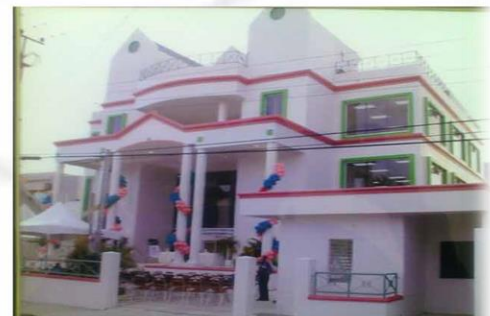
Rebuilt: 57-59 Dundonald Street POS
